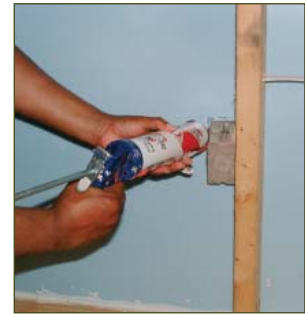
Air sealing with caulk around an electrical
